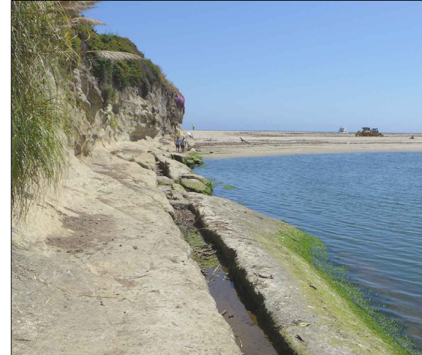
D TYPICAL (E) TRENCH CONDITIONS PHOTO DETAIL - LOOKING SOUTH
