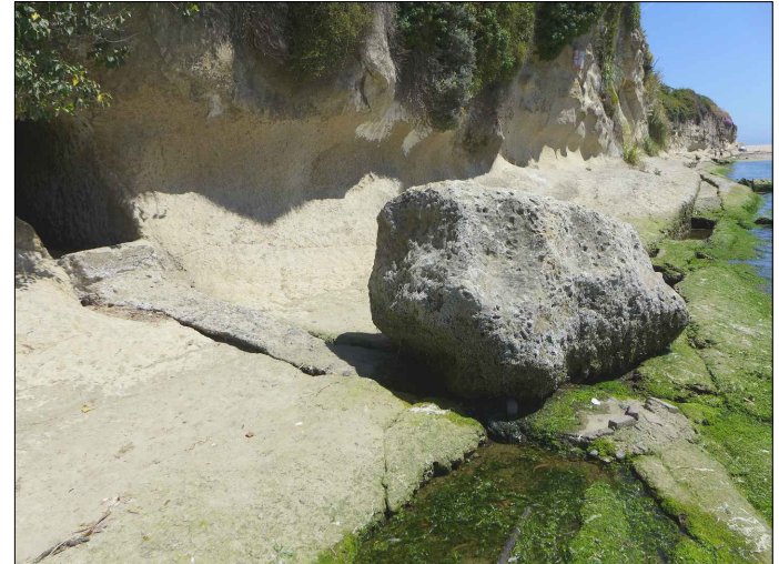
A TUNNEL OPENING AND BOULDER NEAR (P) JUNCTION BOX PHOTO DETAIL - LOOKING SOUTH
