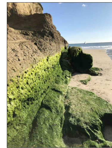
F TYPICAL (E) TRENCH CONDITIONS PHOTO DETAIL - LOOKING SOUTH
