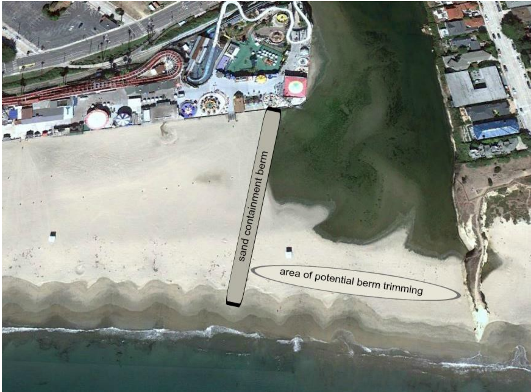
San Lorenzo River Culvert Project (Corps File No. SPN-2014-00434)
